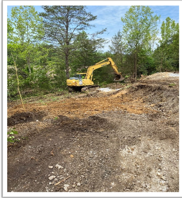
Photo 4: Kentucky Processing and Bowie Refined Coal, PCB contaminated soil excavation.
