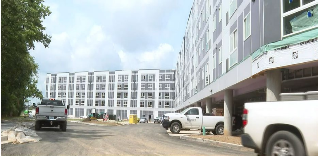
Photo 9: Apartments under construction at 330 Newtown Pike, Lexington, KY
