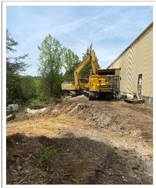
Photo 5: Kentucky Processing and Bowie Refined Coal, PCB contaminated soil excavation.
